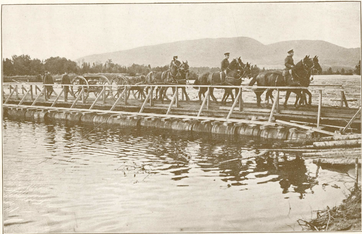
7th Battery Field Artillery (St. Catharines) crossing Pontoon Bridge. This bridge is 300 feet long and was built by the Engineering Corps in 4 hours. This is a new record for the distance.
